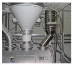
The majority of conveying tasks for pneumatic Volkmann vacuum conveyors are for capacities between 10 and 6000 kg/h (**Figure 4**) whereas under extraordinary circumstances occasionally up to 16 t/h can be reached. Distances vary from just a few meters to up to 100 horizontal and up to 40 meters vertical.
