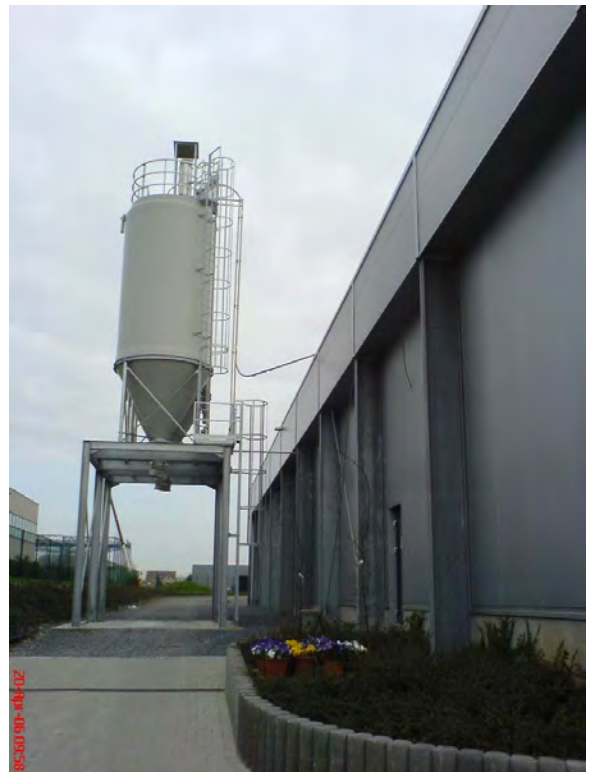
Fig 6 Total elevation of 50 feet in two sections
