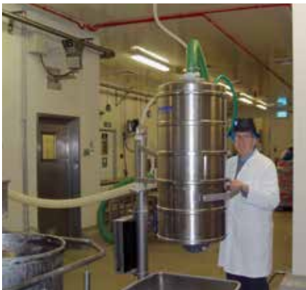
Flour transfer system in a bakery.
