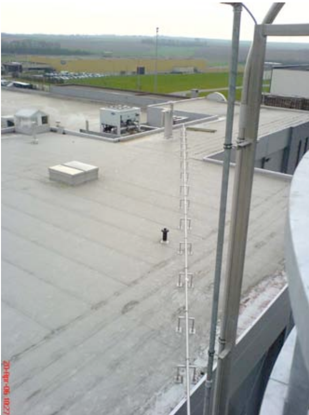
Fig 5 Long Horizontal Conveying Run
